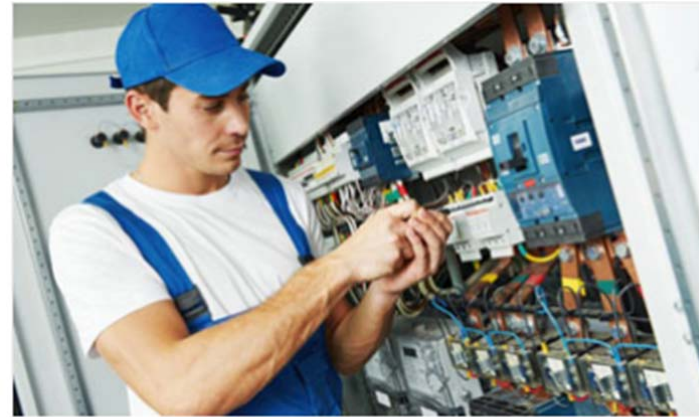
Electrical Maintenance Service
